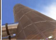
As part of a major refurbishment, **Brocklebank 20/3** decorative wire mesh cladding was added to the concrete chimney stacks at Pulrose Power Station, Isle of Man.
