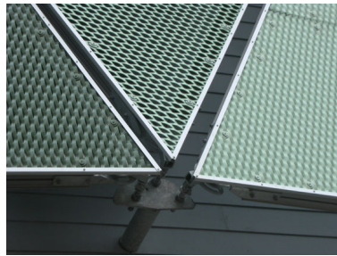
Garston architectural expanded metal installed as rain screen cladding at Carnegie Pavilion, Headingley Cricket Ground, Leeds, England.
