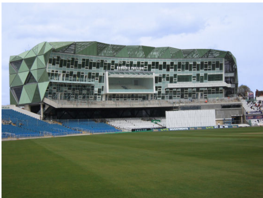
Garston architectural expanded metal installed as rain screen cladding at Carnegie Pavilion, Headingley Cricket Ground, Leeds, England.
